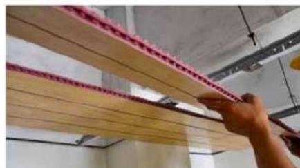
05 Fix the acoustic panel together one by one
