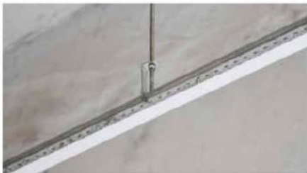
01 Fix the tee grid system onto the ceiling
