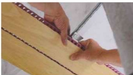
04 Fix the WY-GA03 clip onto acoustic panel
