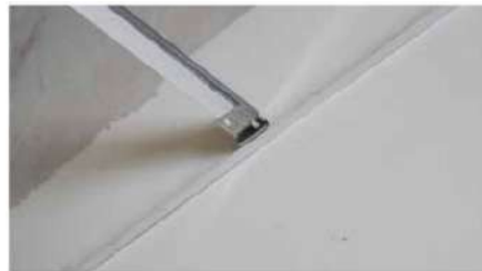
02 Fix the WY-GA02 clip onto the tee grid
